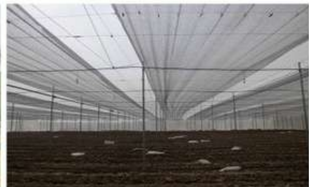
FLAT ROOF TYPE NET HOUSE WITH WIRE ROPE CONSTRUCTION
